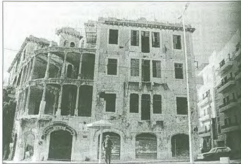
In 2002, a significant number of buildings in central Beirut, Lebanon, remained in a state of total disrepair, a visual reminder of the intermittent war that engulfed the country for more than two decades.
